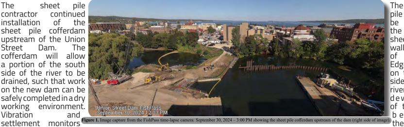
were closely observed during sheet pile installation and pile wall and auxiliary spillway will begin shortly so the new no thresholds have been exceeded. The upstream portion spillway can be installed. Work has also begun on a temporary of the sheet pile cofferdam is nearly complete (Figure 1). crane platform below the Union Street Dam to begin work on the downstream portion of the sheet pile cofferdam.
